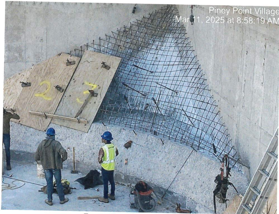
Top portion of rebar NW corner.
