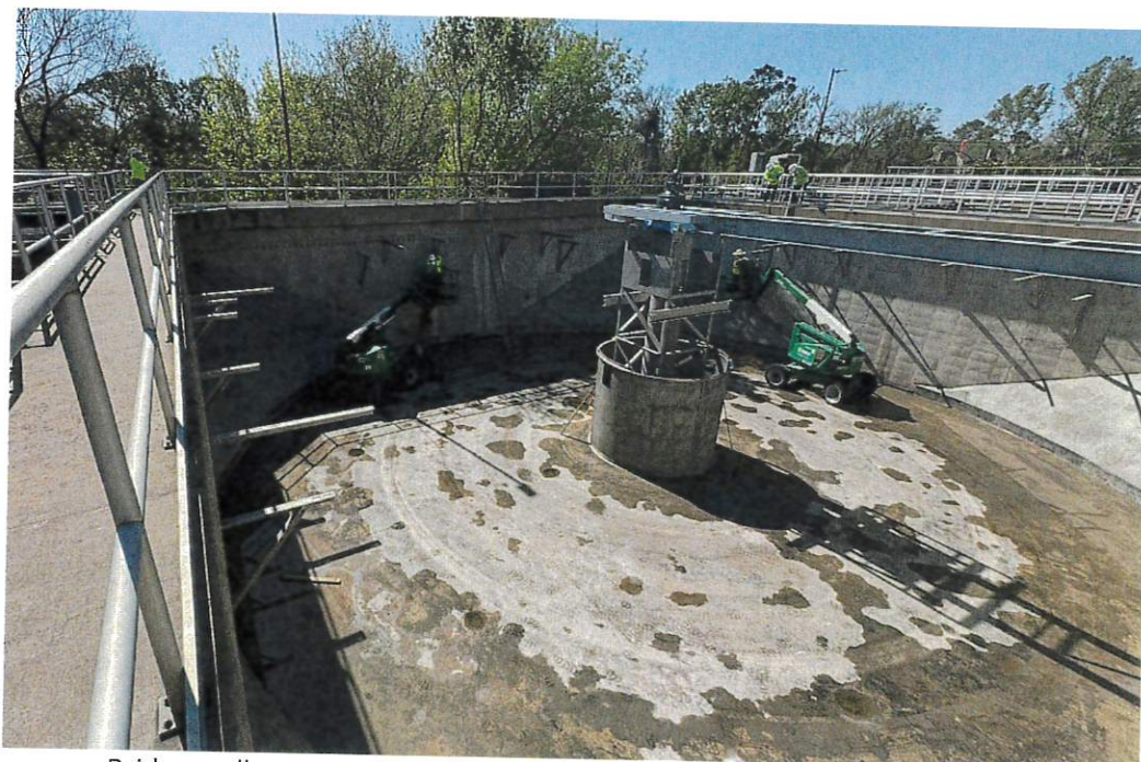
Bridge walkway, center pier, influent well, and effluent trough supports.
