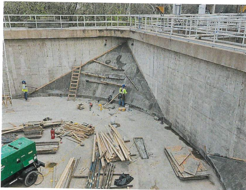
Wrecking forms for SW corner.
