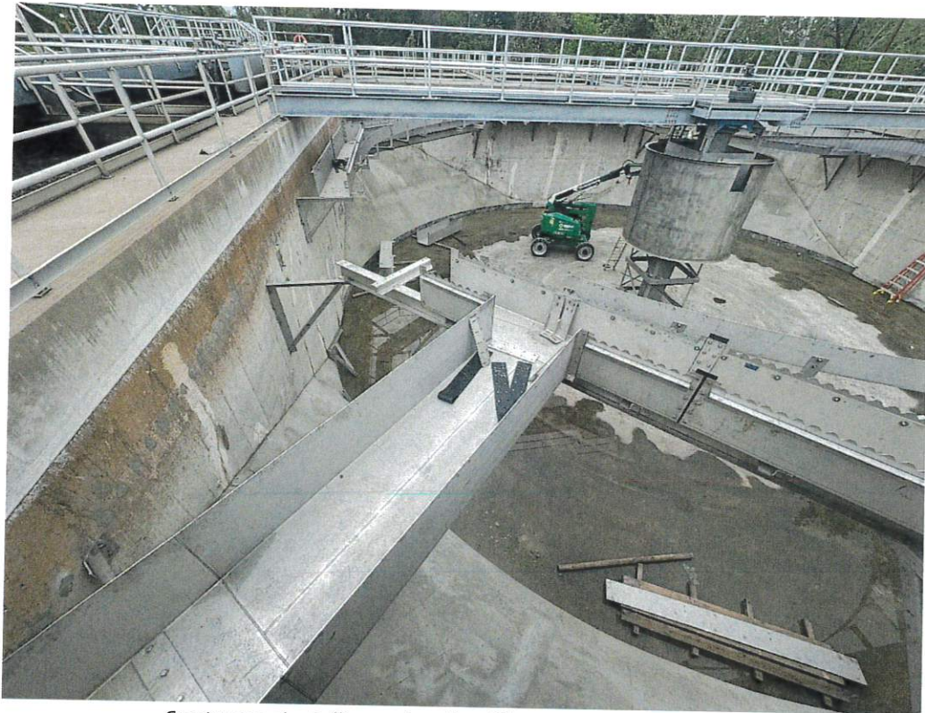
Contractor installing catwalk, effluent troughs and weirs.
