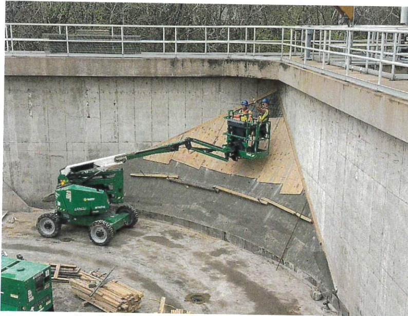
Setting formwork for SW corner of clarifier.
