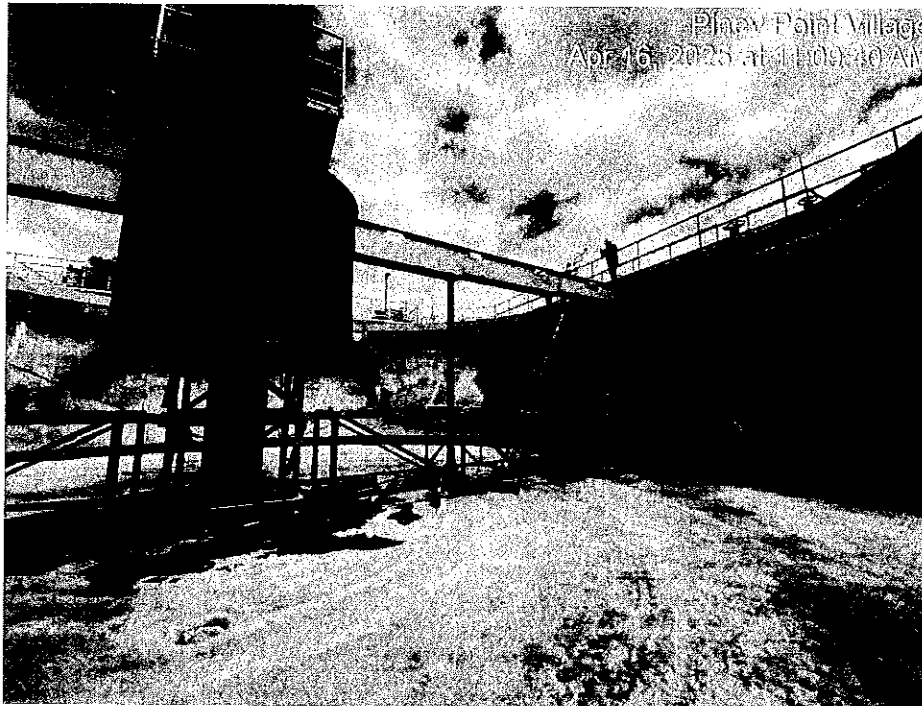
(4/16) – Interior of Clarifier from Final inspection walkthrough.
