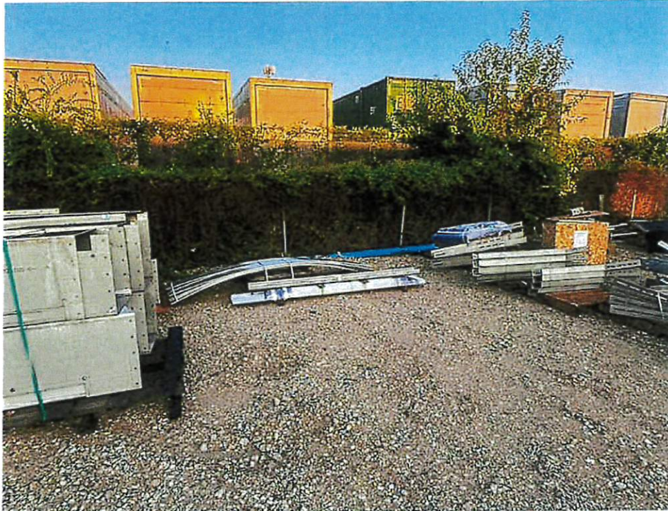
(9/2) – The Contractor has received Effluent Trough and Scum Baffle Materials at their yard.
