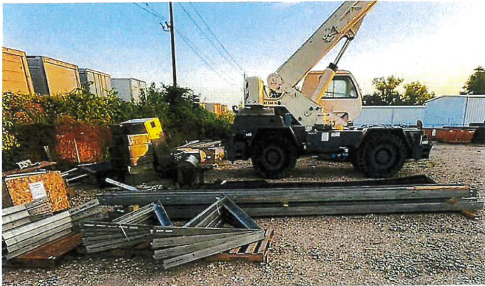
(9/2) – The Contractor has received Effluent Trough Materials at their yard.
