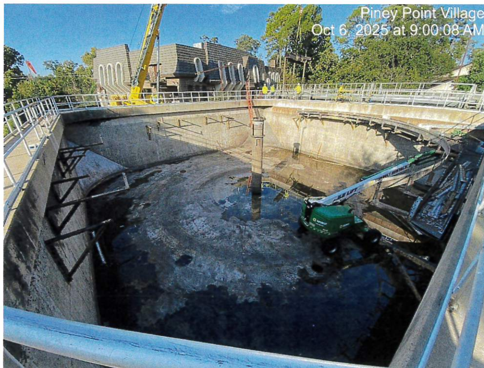
(10/6) – Demolition of the existing interior clarifier mechanism continues.
