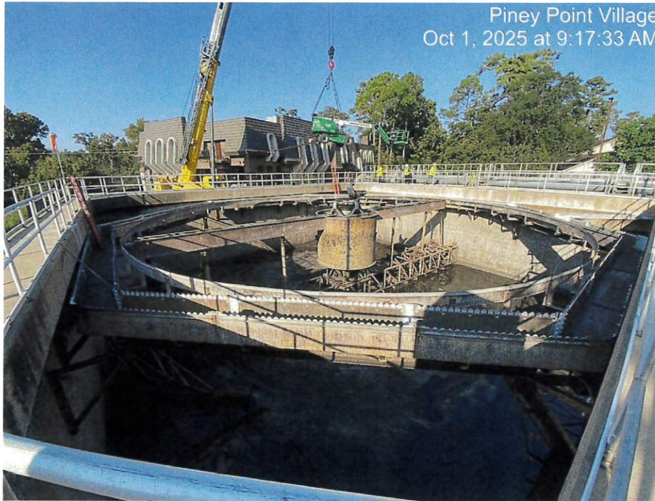
(10/1) – Demolition of the existing interior clarifier mechanism proceeds.
