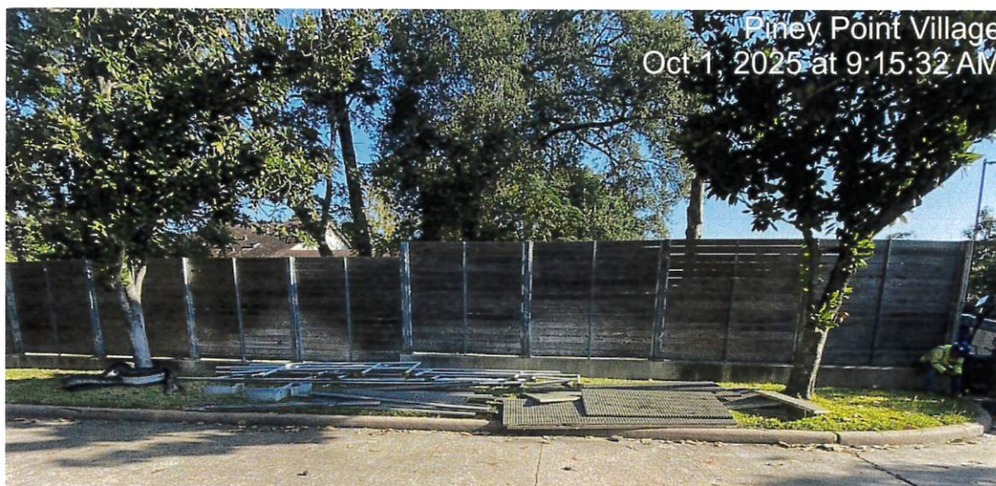
(10/1) – The existing bridge, handrails and grating were removed.
