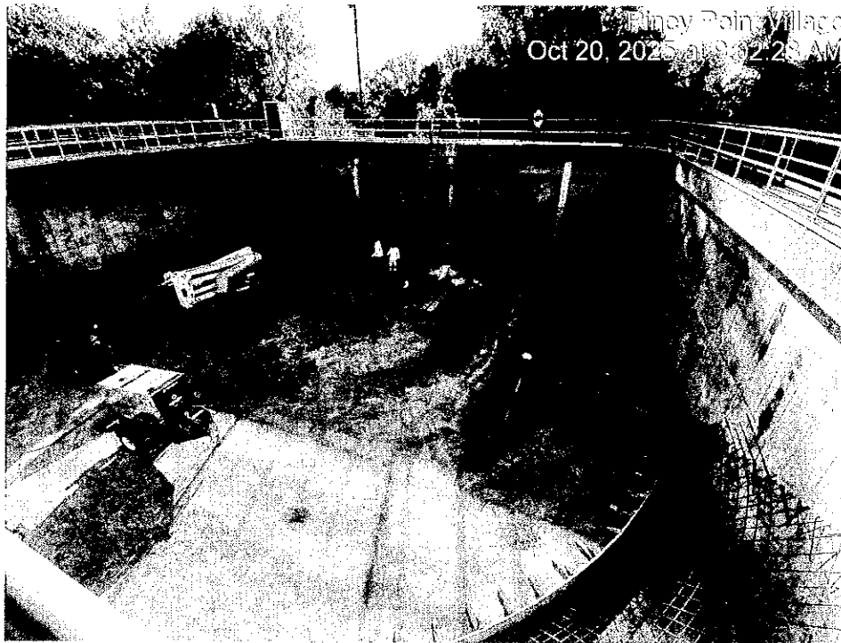
(10/20) – Corner rebar reinforcement, and grout ring placement continues.
