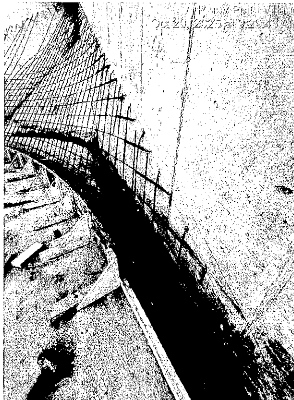
(10/20) – Corner rebar reinforcement, and grout ring placement continues.
