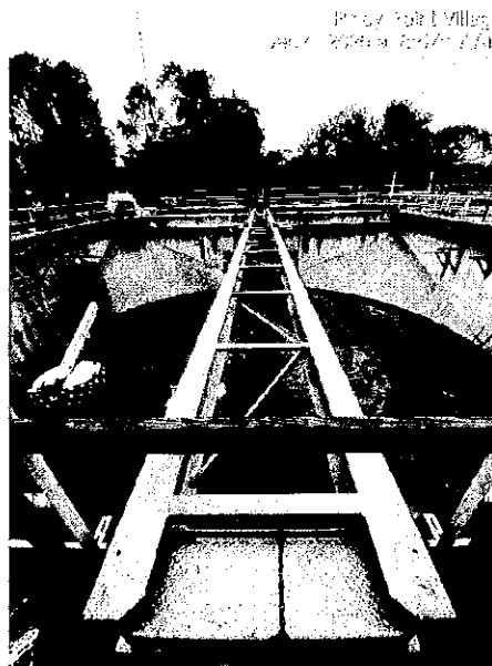
(12/4) – Contractor preparing to install grated walkway.
