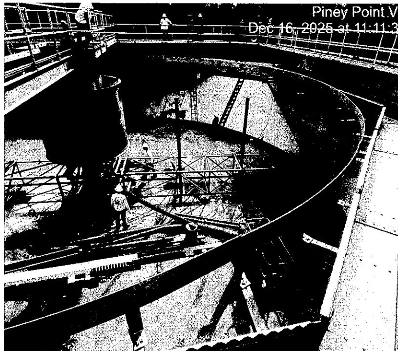
(12/16) – Contractor continuing the construction of the truss rack arms.
