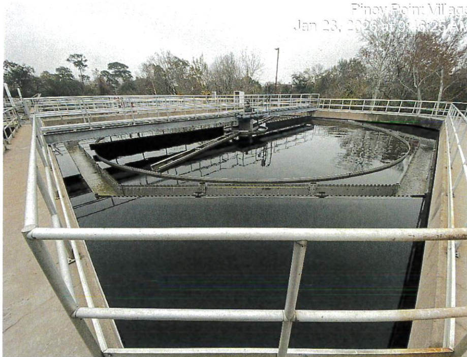
(1/23) – Construction of South Clarifier is complete
