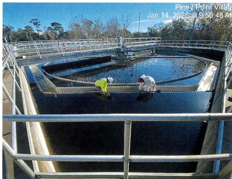
(1/14) – Contractor making final weir adjustments.
