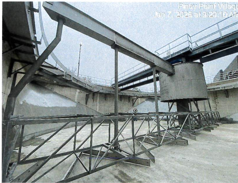
(1/7) – Walk-Thru Inspection of South Clarifier.
