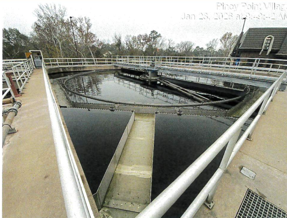
(1/23) – Construction of South Clarifier is complete
