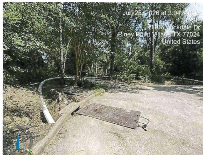
(6/25) – Contractor proceeds with pipe-bursting the 1 st line segment along Wickdale Dr., starting at the end-of-line cleanout located at the end of the cul-de-sac.
