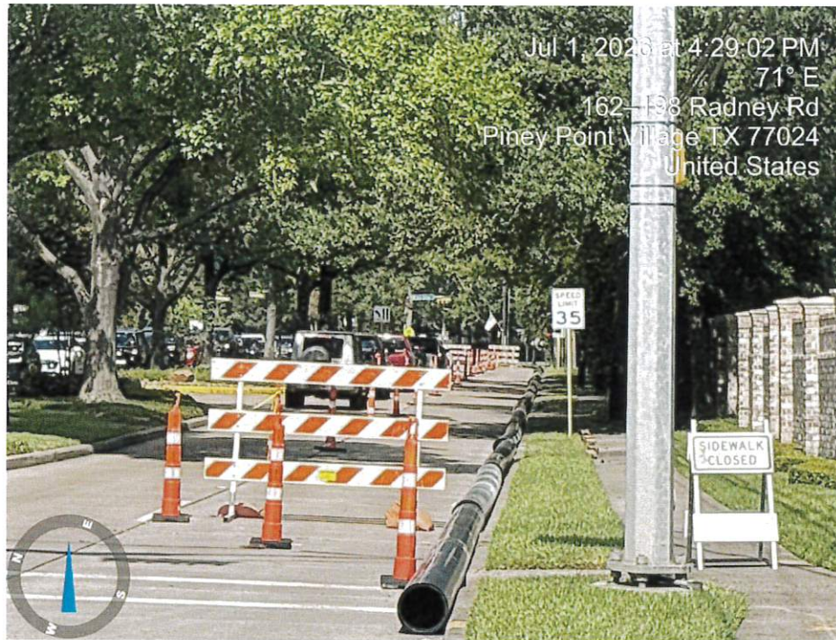
(7/1) – Staging by-pass lines within traffic control
