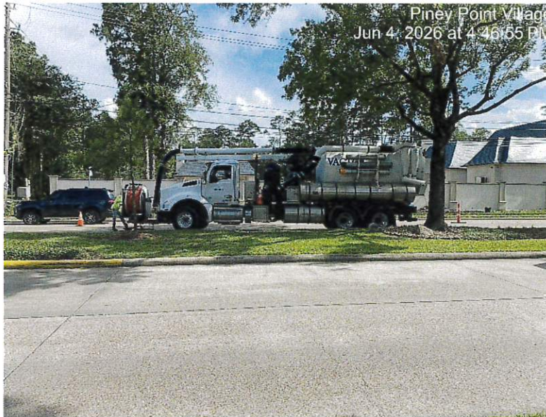
(6/4) – Contractor performing sanitary sewer cleaning
