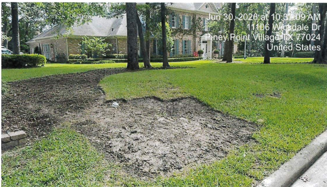
(06/30) – Contractor prepares for sod restoration following service reconnections along Wickdale Dr.
