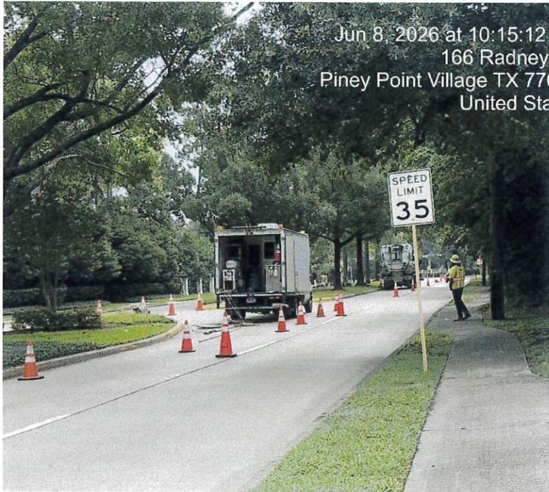
(6/8) – Contractor performing cleaning and televising within traffic control
