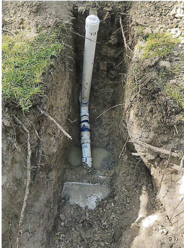
(6/26) – Contractor proceeds with service reconnections following pipe-busting operations along Wickdale Dr.
