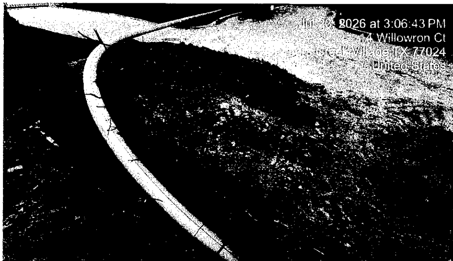
(7/23) – Contractor proceeds with pipe-bursting along Willowron Ct.
