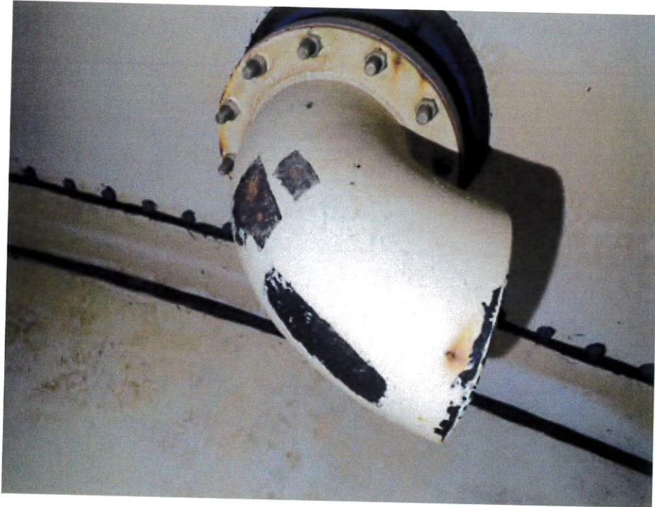
Staining was noted on the well fill line with apparent coating failures.
