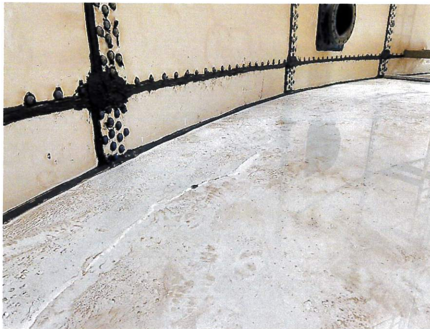
Additional GST concrete floor failures were noted.
