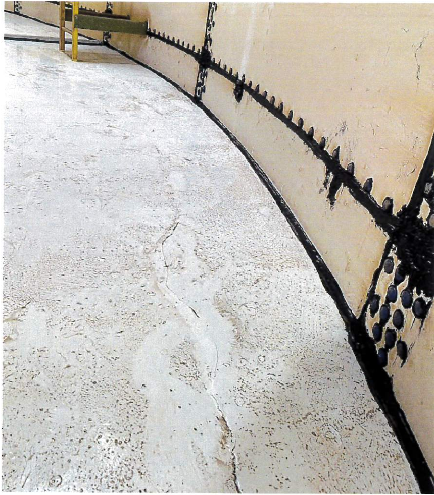
Additional GST concrete floor failures were noted.
