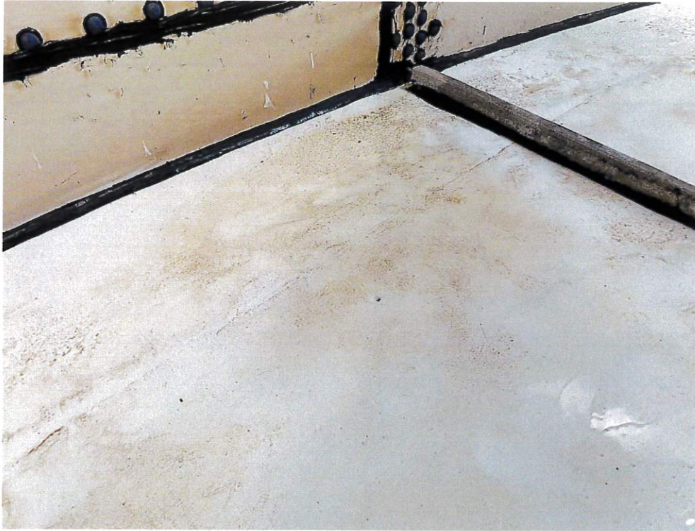
Previously repaired GST floor sections appear to be holding up well.
