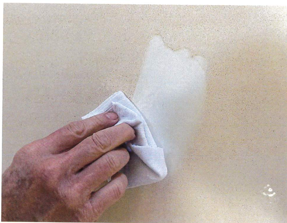
Sidewall interior coating appears to be in excellent condition.
