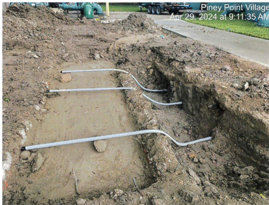
Installed electrical conduit for proposed booster pumps.
