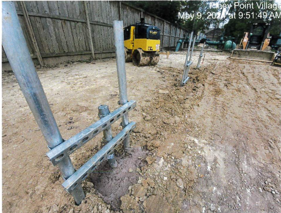
Installed electrical stub-ups for proposed booster pumps.
