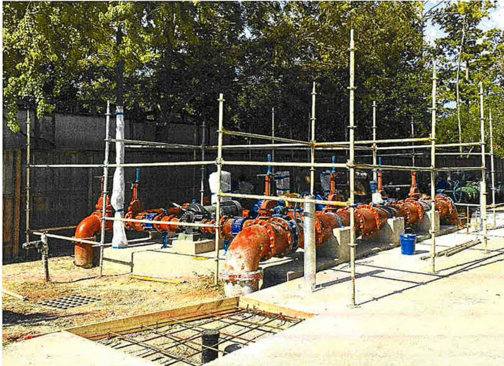
(8/21) – Installation of scaffolding, in preparation of sand blasting and coating of new booster pump piping and valves.
