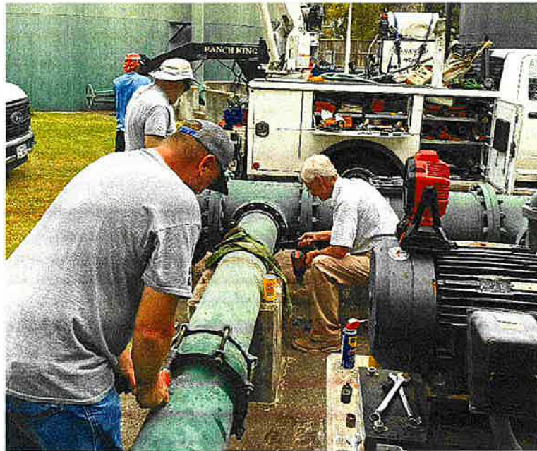
(8/20) - Existing header piping, downstream of the existing Pressure Relief Valve (PRV), being modified to allow improvements to the existing PRV.
