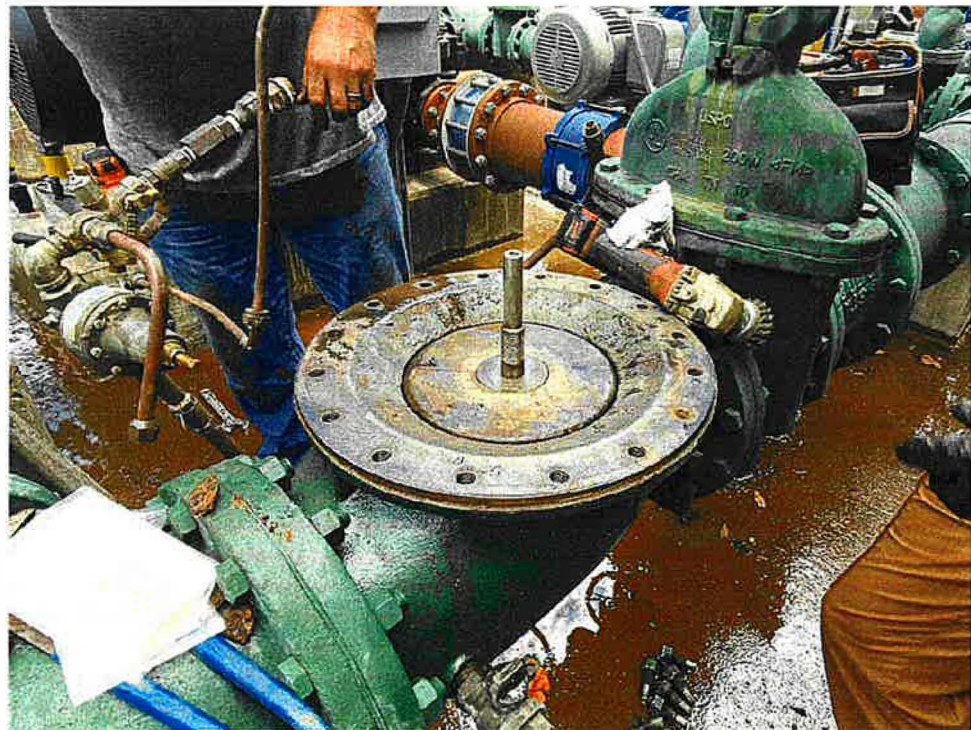
Installation of 10" PRV Internal Disc Retainer Diaphragm, as approved via Change Order No. 3.
