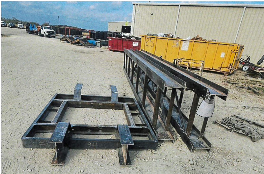
Carbon Steel Access Bridge and Platform are currently at the Galvanizer in Houston and are near completion.
