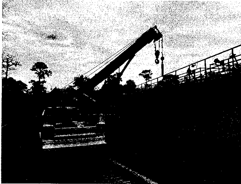
(1/14) – Mobilization of Equipment, Materials, and Personnel to site.
