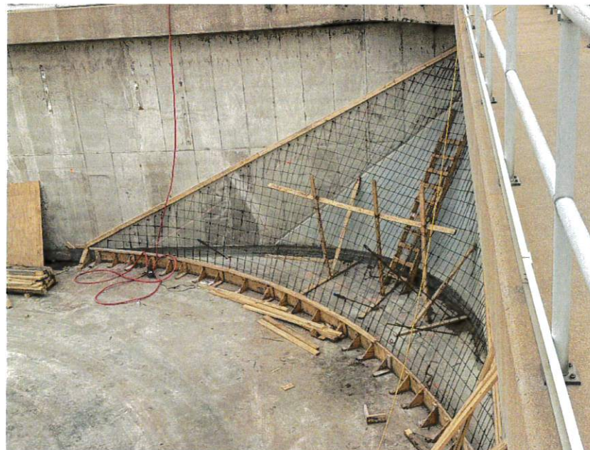
Complete rebar for clarifier corner.
