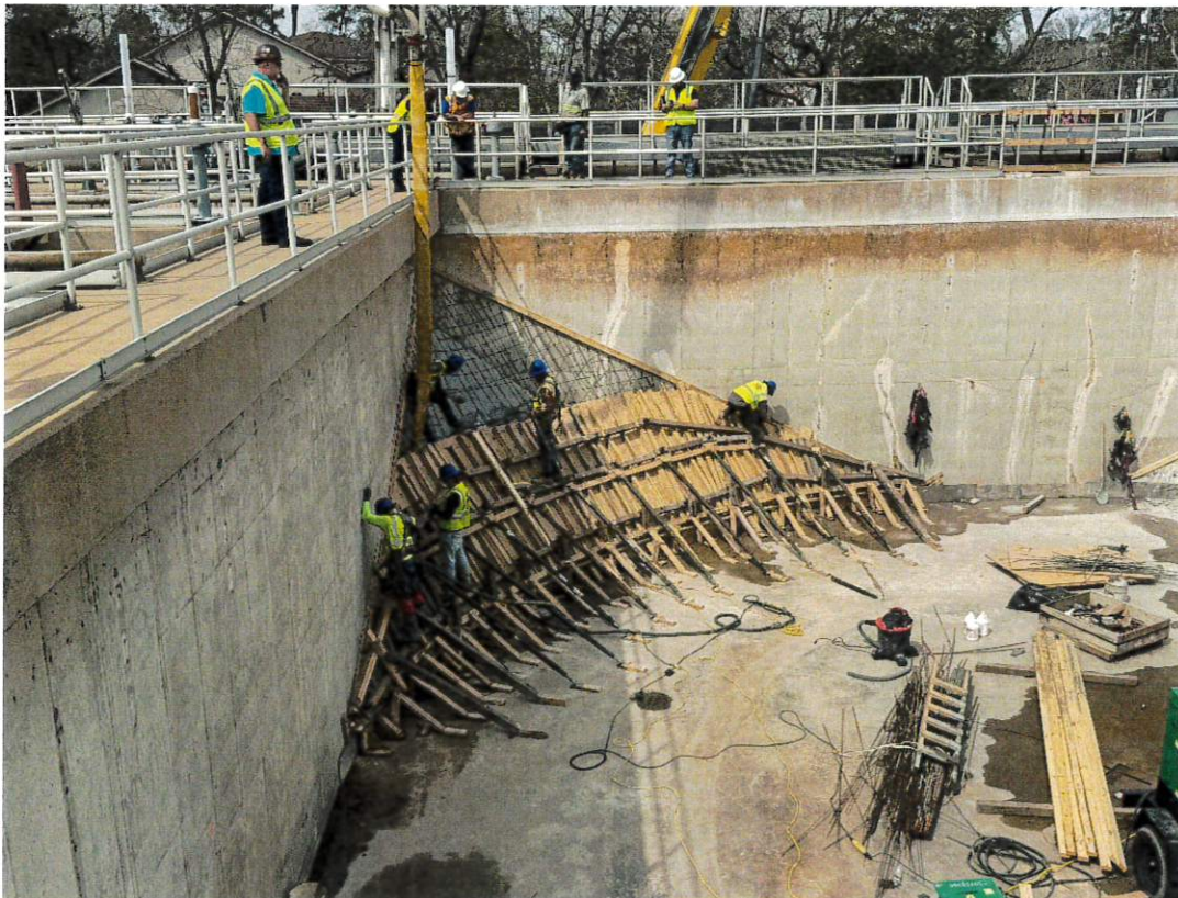
Contractor pumping concrete for the first segment of NW corner.
