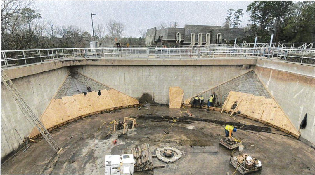
Formwork for NW & SW clarifier corners.
