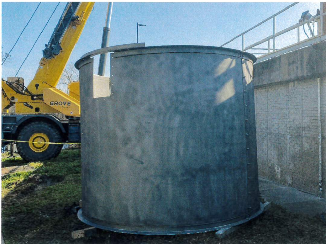
Clarifier Stainless Steel Influent Well Delivered to site, in preparation for installation.
